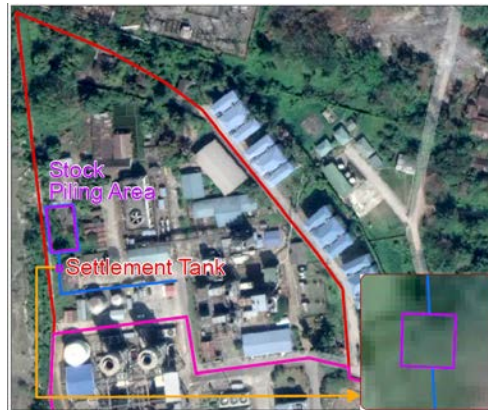
Figure 9-1: Stock piling area at Project site
